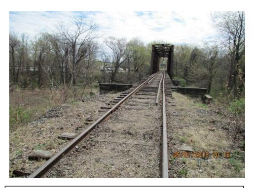
Looking East at the existing U&D Railroad bridge over the Esopus Creek. The existing structure will be rehabilitated for Alternative 2.
